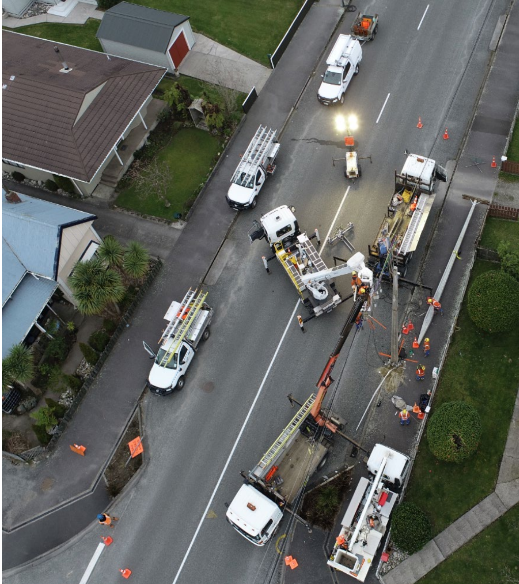
BEL Pole replacement
