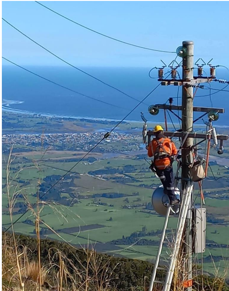
Buller Electricity Lineman working at Mt Rochfort overlooking Westport Township
