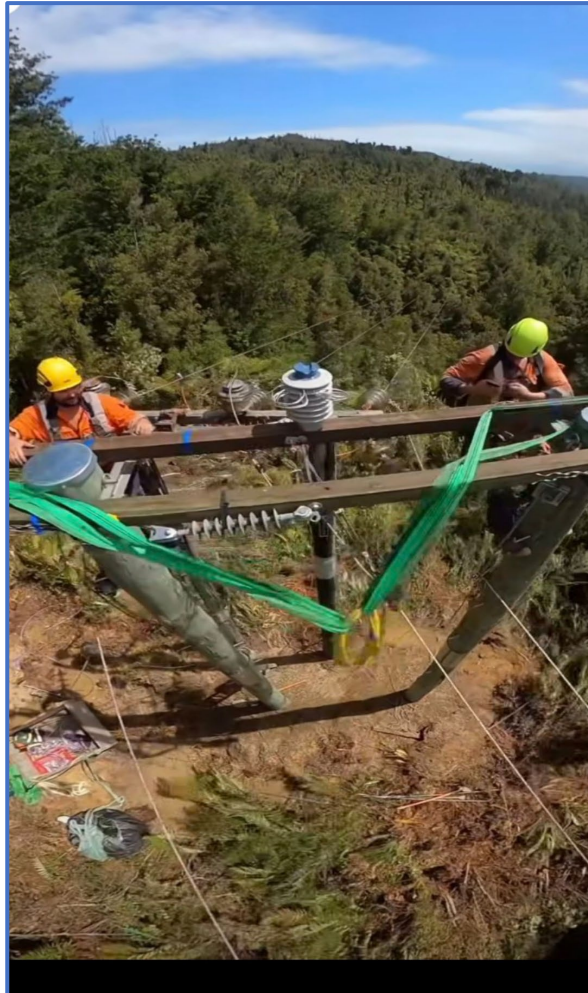
Buller Electricity Linemen working in the Karamea Bluff replacing a 33kV double pole structure via helicopter
